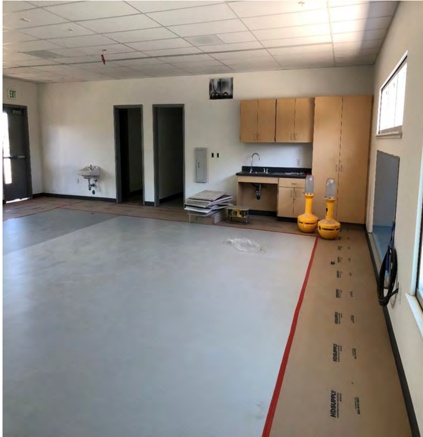
Pre K East Flooring
