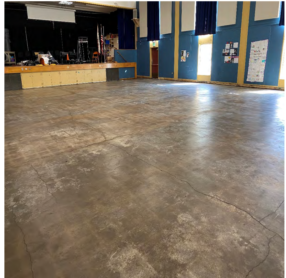
Multi-Use Building Floor Demolition
