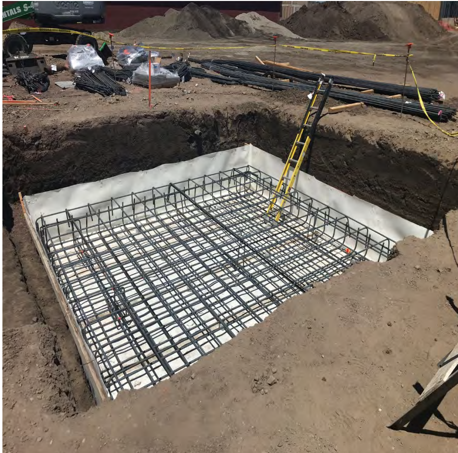
Science Elevator Footing
