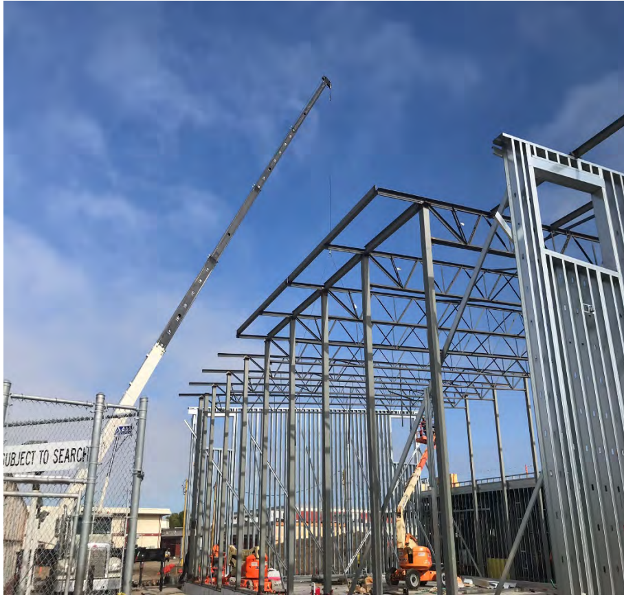
Gym Truss Install
